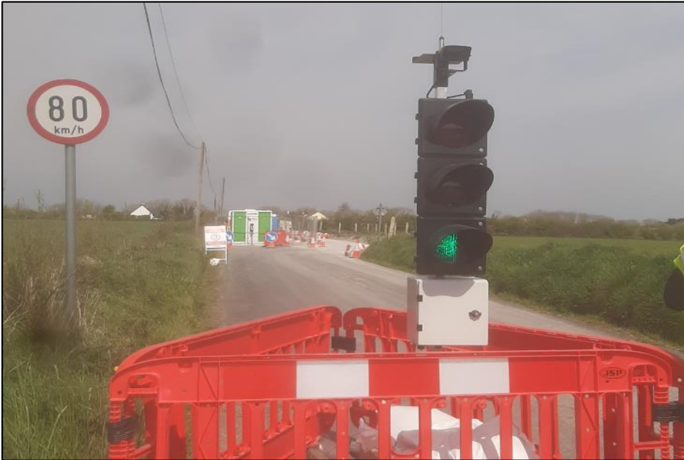
Figure 2.6: Sensor controlled traffic management at operational joint bay location
