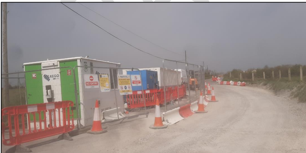
Figure 2.7: Operational joint bay location comprising temporary welfare facilities (green and white cabinet), generator (blue cabinet), jointing bay (white container over joint bay), and associated vehicle. A passing bay allows traffic flow around the joint bay – note natural revegetation of the edge of the passing bay
