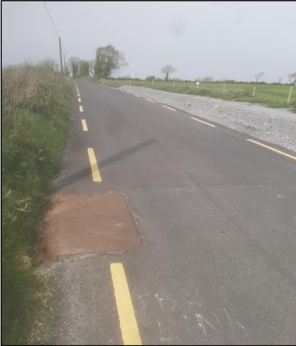
Figure 2.4: Reinstated public road at a joint bay location (darker tarmac on road) with associated fibre optic link box and passing bay, currently dormant and bermed with stone prior to jointing works at the joint bay
