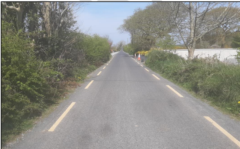
Figure 2.5: Reinstated local public road following the laying of UGC
